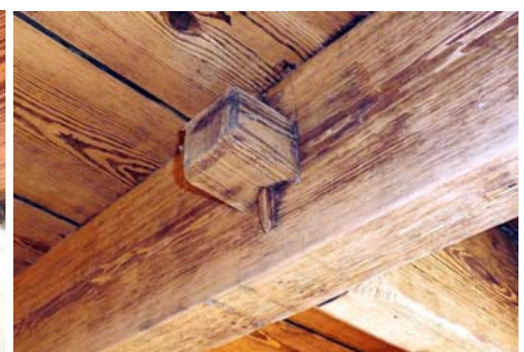
Yellow pine floor joists joined via through mortised technique. Notice the locking wood pin.
