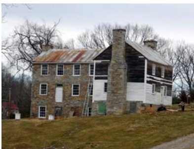
Front portion of the house is log covered in weatherboard - 1790. This view shows both the front and rear section
