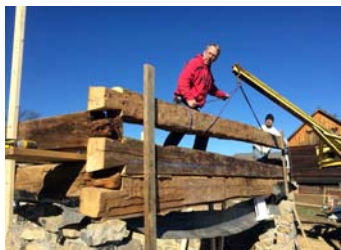
Under reconstruction, note full-dovetailed logs
