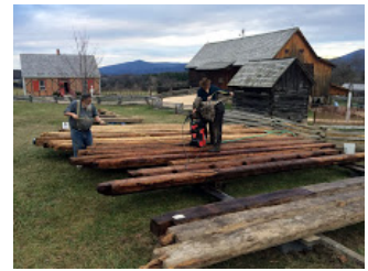
Powerwashing original logs prior to storage
