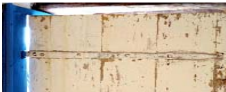
Hand forged strap hinge, possibly original 18th century
