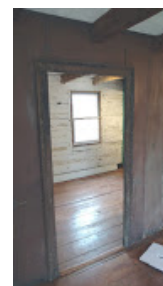
1st floor as reconstructed, note single panel wall
