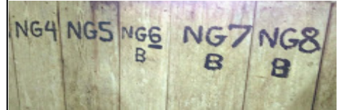
2nd floor walls showing numbering scheme
