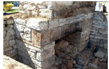
Cellar cooking fireplace before disassembly
