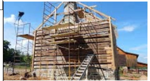
Under construction, original logs all numbered with minor repairs
