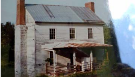
North side, once rear entry, before restoration
