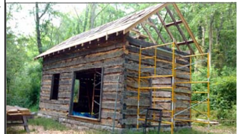
Old log building on Watkinson property being reconstructed for a workshop.
