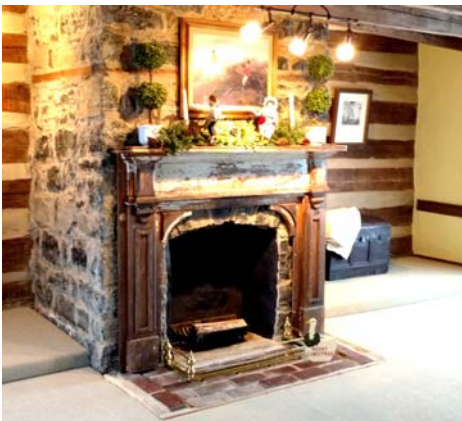
Large second floor fireplace sharing chimney with first floor double fireplaces
