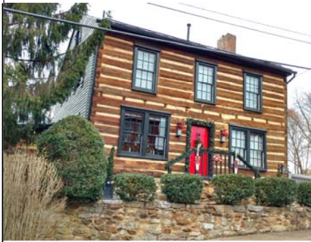
Front View - Earliest portion of house
