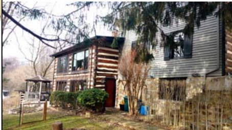
View of the south side showing addition constructed of reused logs
